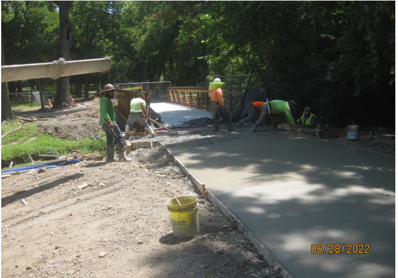
➤ 120' bridge at Dixon Branch is installed, and deck is poured.
